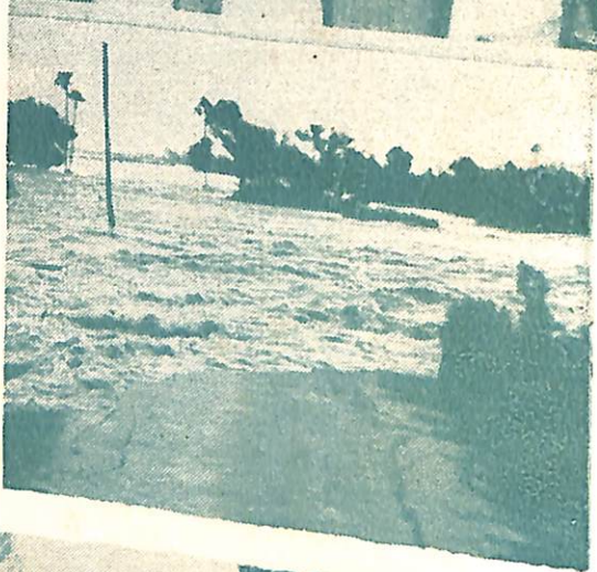
A breach on the Bhalukhai embankment and mad rush of flood-water (Cuttack district)
